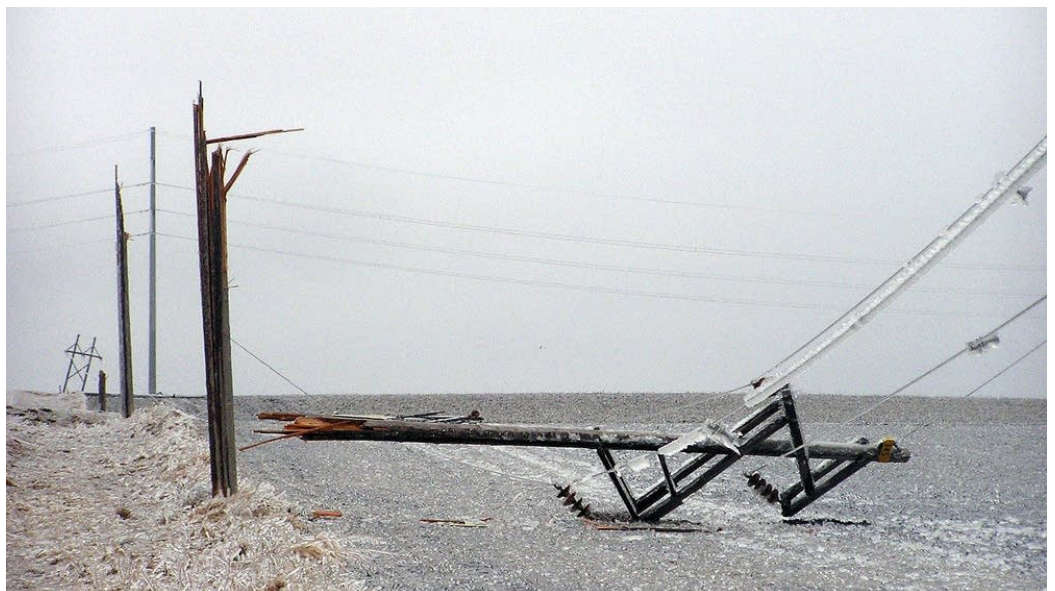
Powerlines down in Worthington, Minnesota (Mark Steil, 2013)
