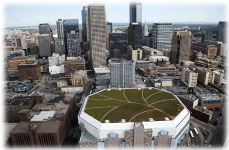
Figure 12: Target Center Green Roof in Minneapolis, MN
